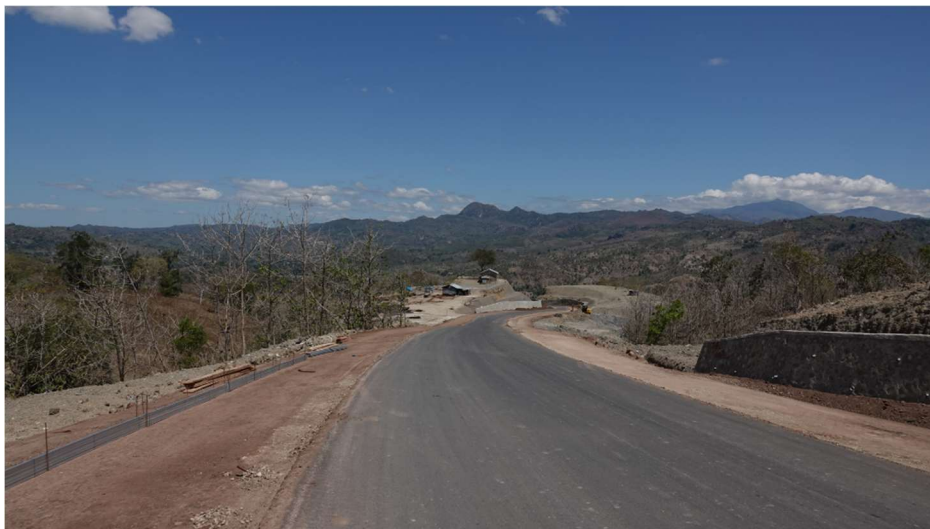
Figure 4. Jalan Sabuk Merah (Red Belt Road) along the Oecusse international border (2024)
